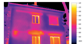
Thermal image with ScaleAssist
